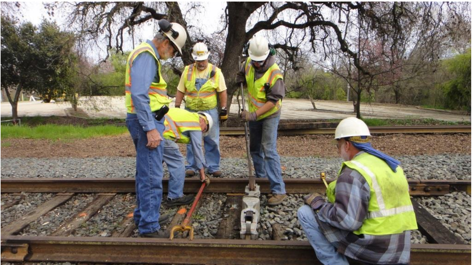
Steve cranks on the track-jack spreading the rails as Alan and the three Mikes keep a close eye on the gauge measurement
