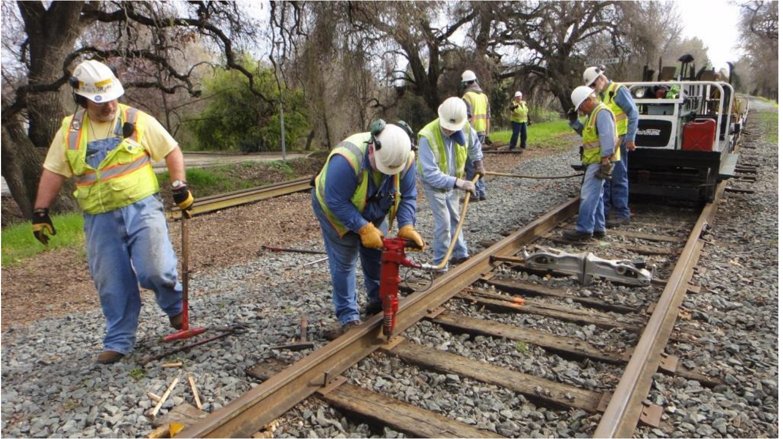
Once the track was gauged correctly, Frank decides that power tools are more efficient and drives spikes with the pneumatic spike-driver
