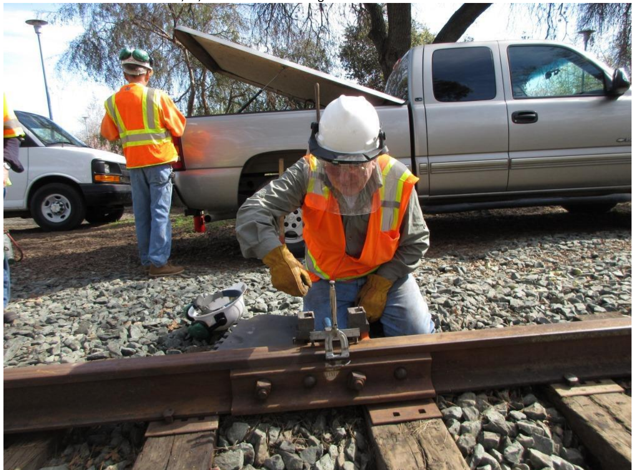
"Locked and loaded!" Joe "Two-Drops" prepares to ignite the thermite catalyst in the Cadwell mold
