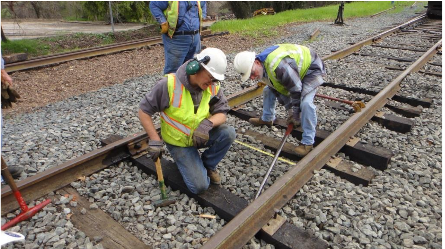
Bent spike? No problem. Mike M. uses the handle end of a claw-bar to bend the spike back away from the web of the rail
