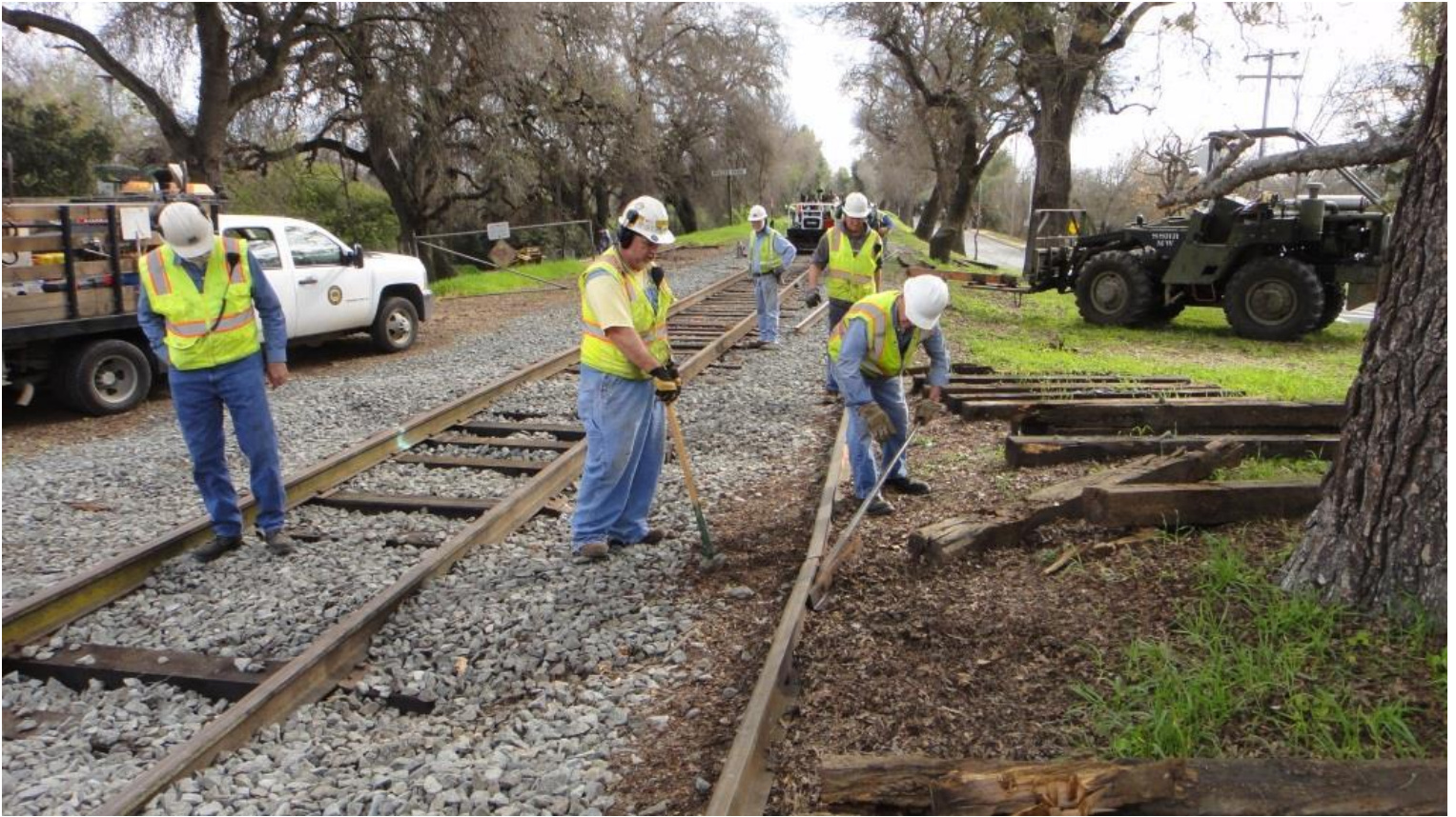
Once loose, Mike T. pries the joint-bars off with a lining bar
