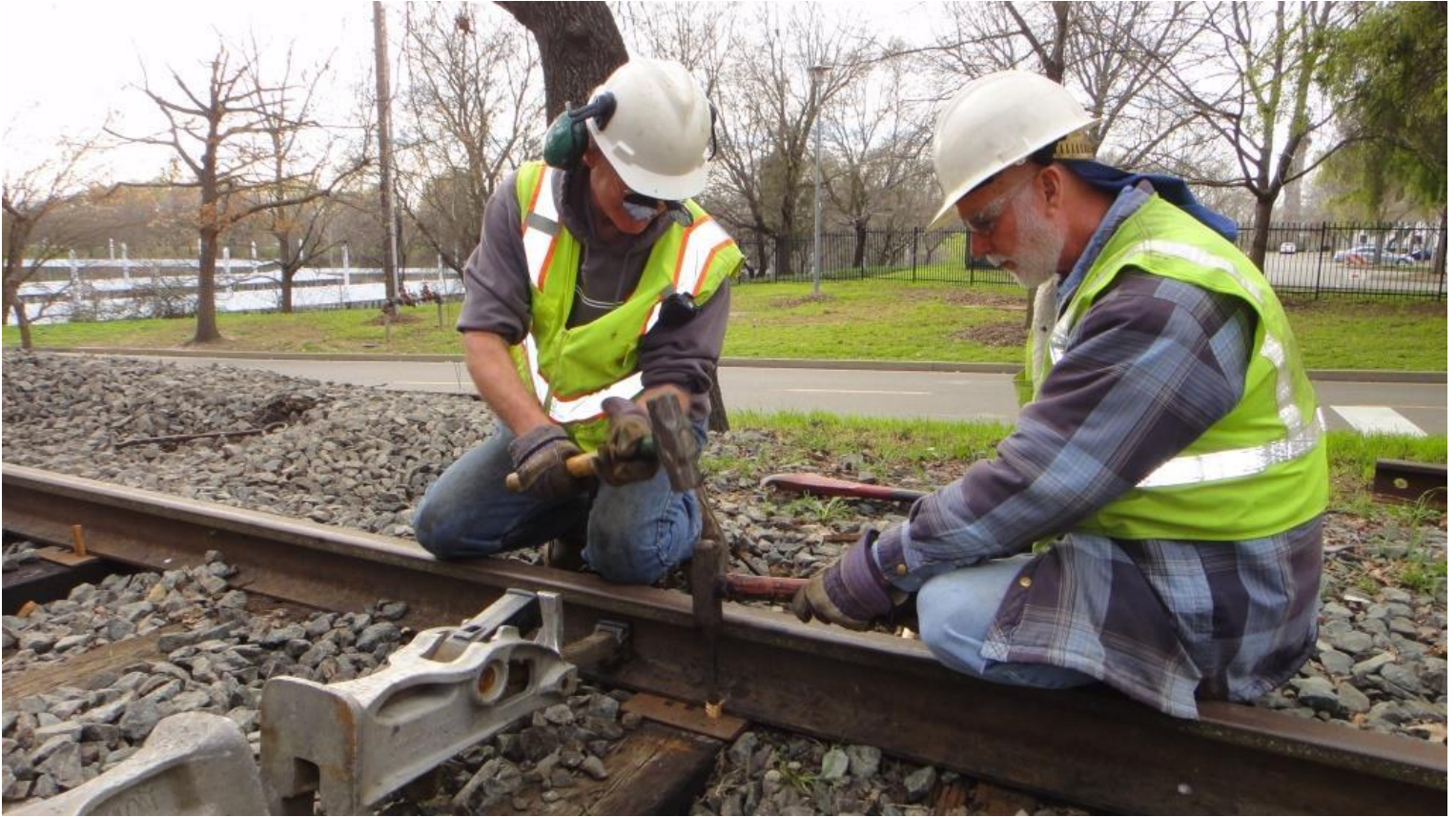
Steve and Mike M. plug old spike-holes in the tie
