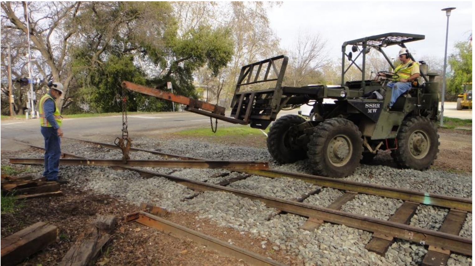
Stage 2 of the operation begins with Mike F. in Big Green removing a stick of the old 75-pound rail with Alan as his guide from the ground
