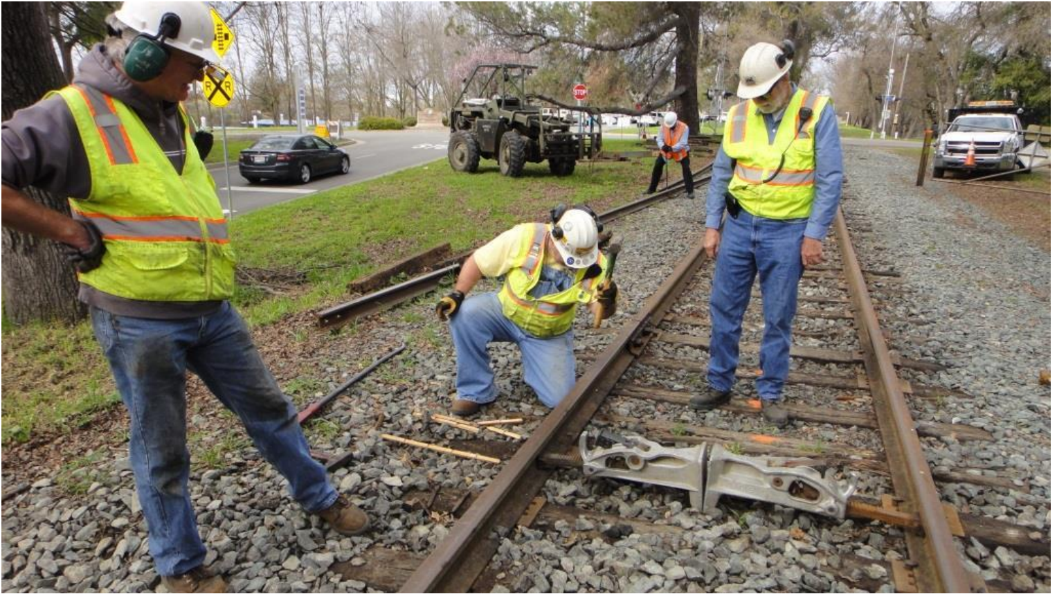
Then, Mike F. employs the one-handed method for setting spikes
