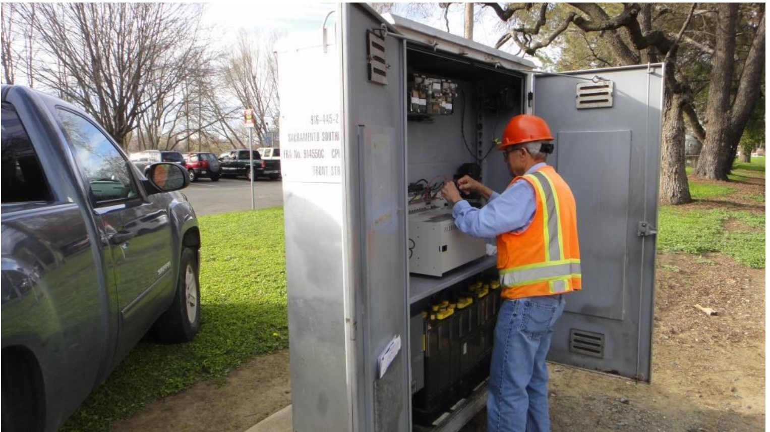
With the MOW Team's departure from the scene, Dale returns the Front Street Grade Crossing Warning System to service
