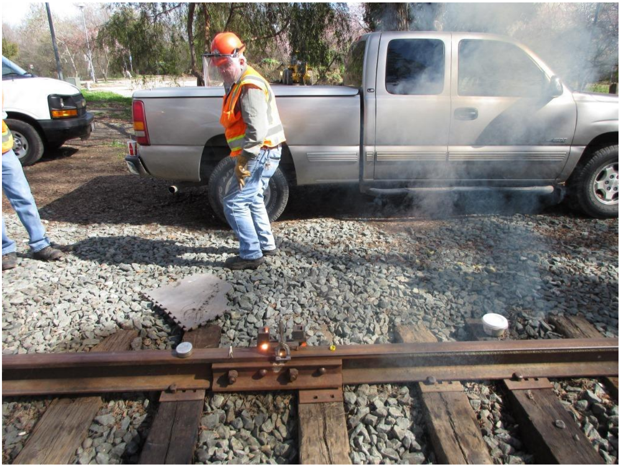
Exothermic welding produces the heat equivalent of lava from a volcano. Wisely, Joe steps away...
