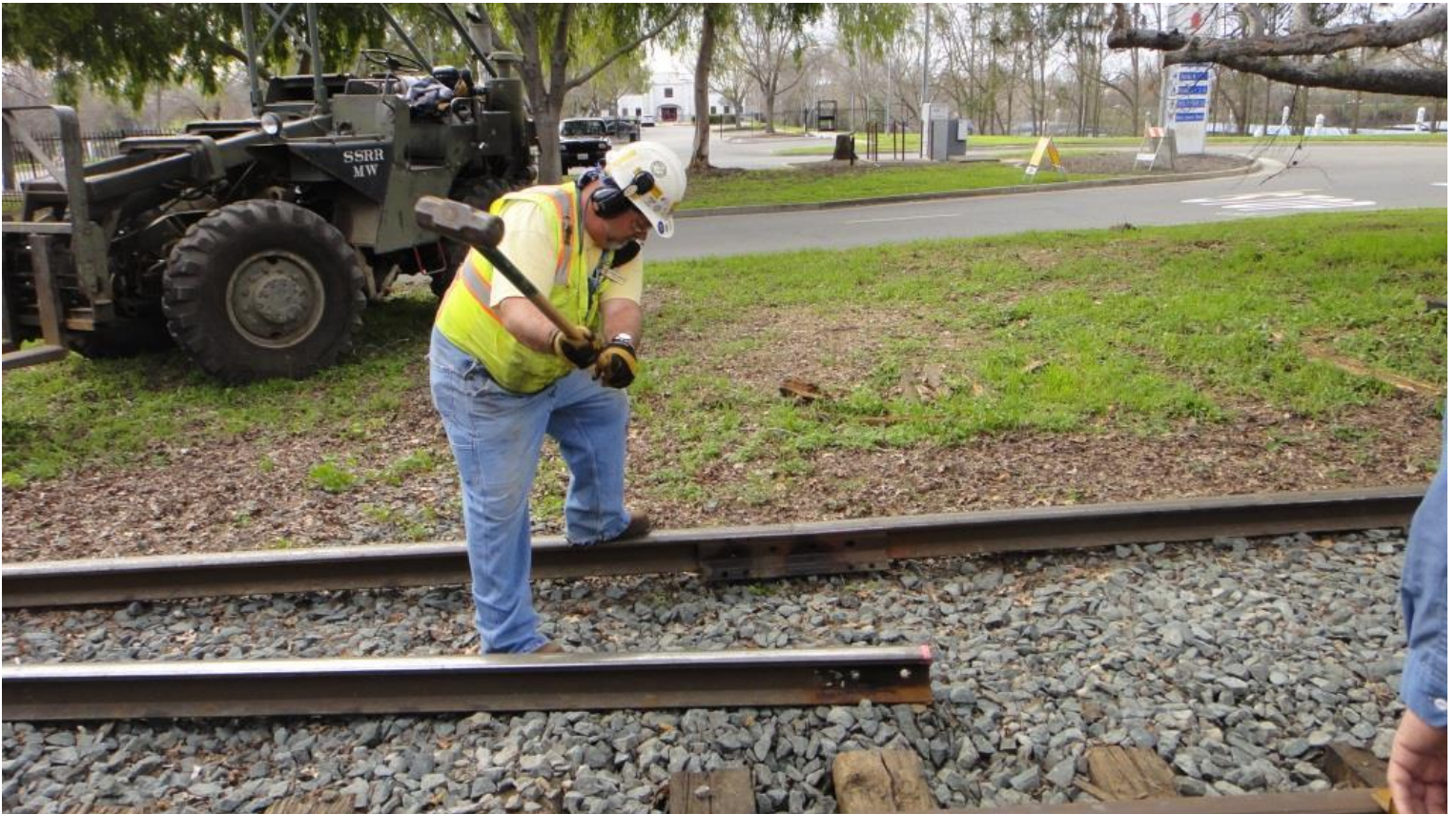
Mike F. uses the whacker-tool to loosen a joint-bar on the old 75-pound rail by giving it a whack
