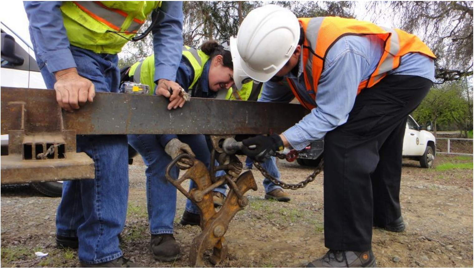
Heather and Jose secure the rail-tongs on the stinger for travel back to the Shops
