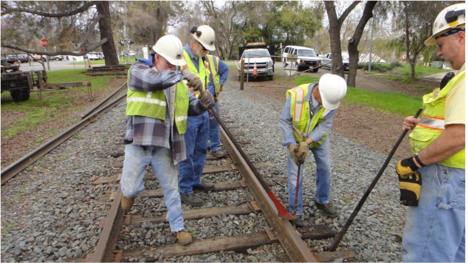
Mike M. and Mike T. employ the “road-master” tool to help provide better leverage for pulling a rather stubborn spike
