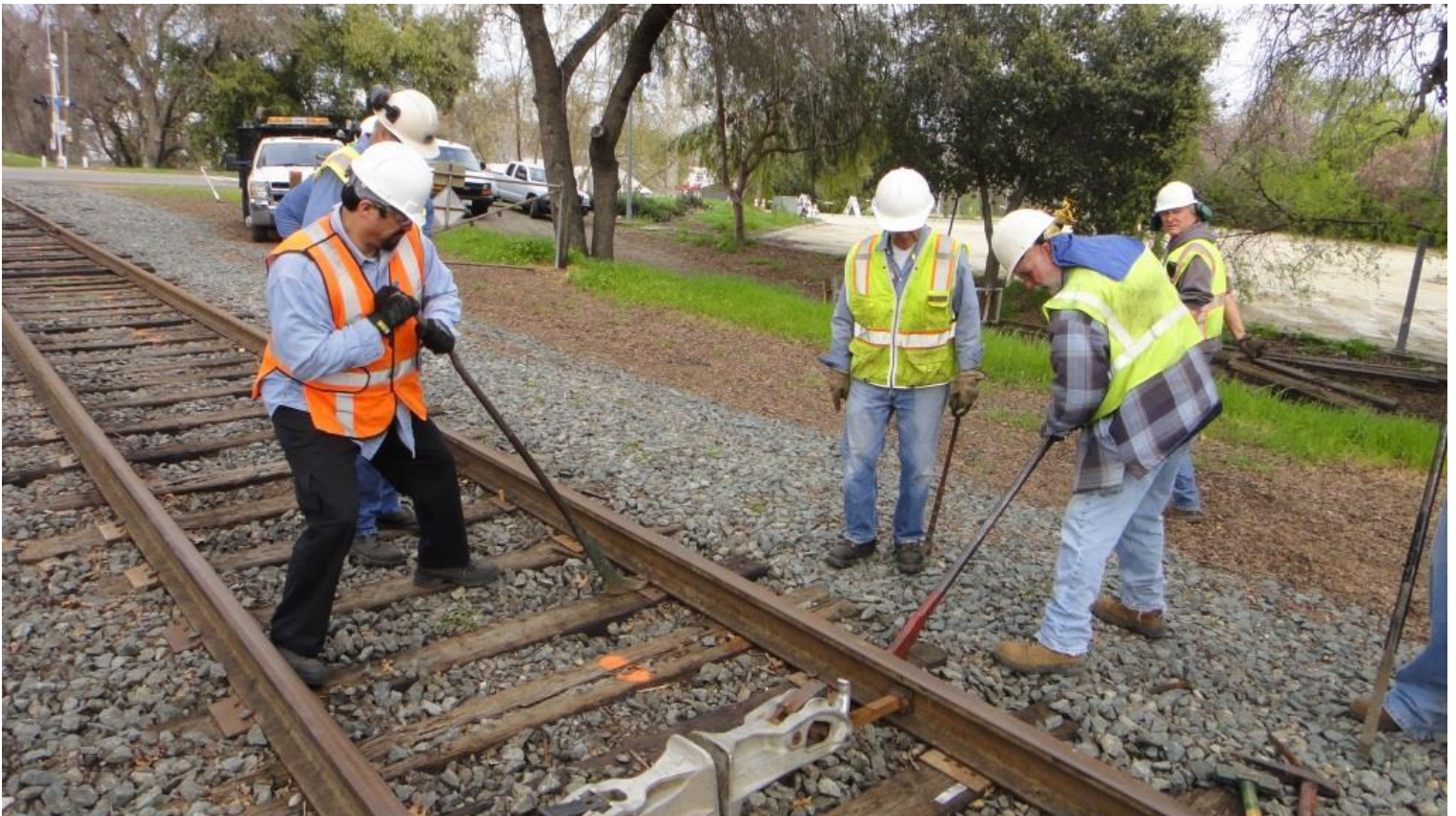
Jose and Mike M. team-up to pull the remaining spikes in the narrow area
