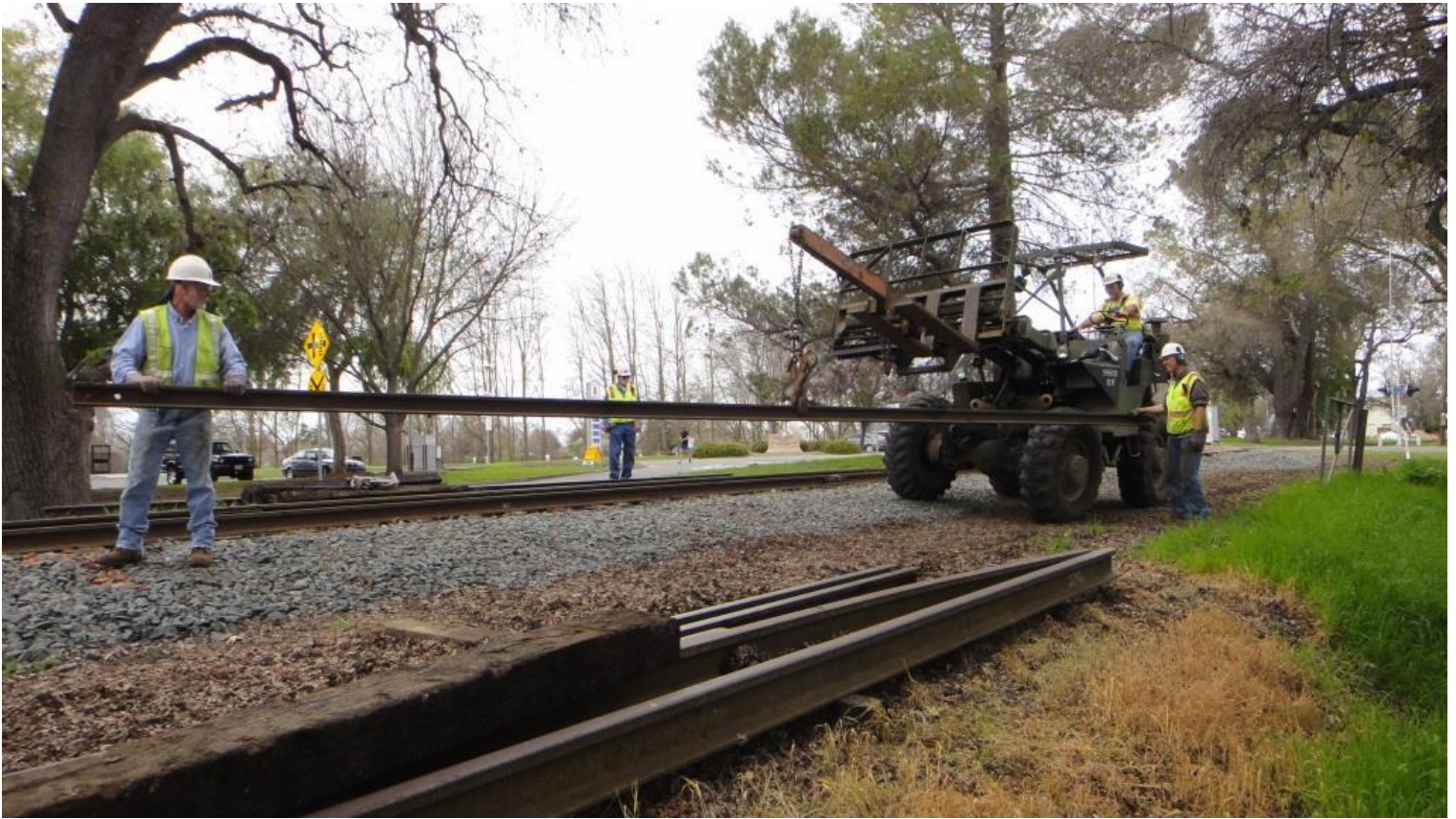
Mike M. and Steve guide a half-ton stick of rail hanging from a chain off the stinger of Big Green
