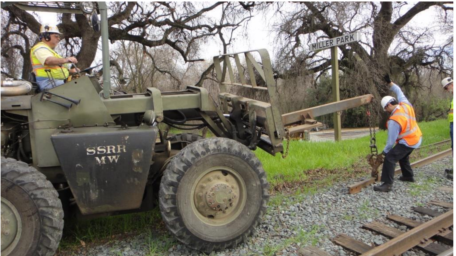
Jose signals to Mike G. on Big Green to lift the next stick of rail
