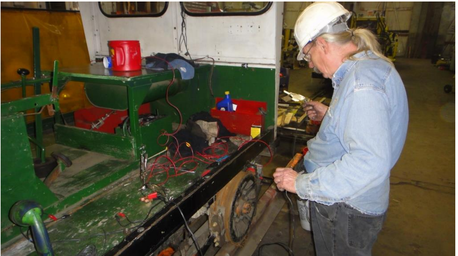
Fred wiring-up the A-4 motorcar so that it will "shunt" the track and trigger the grade-crossing systems
