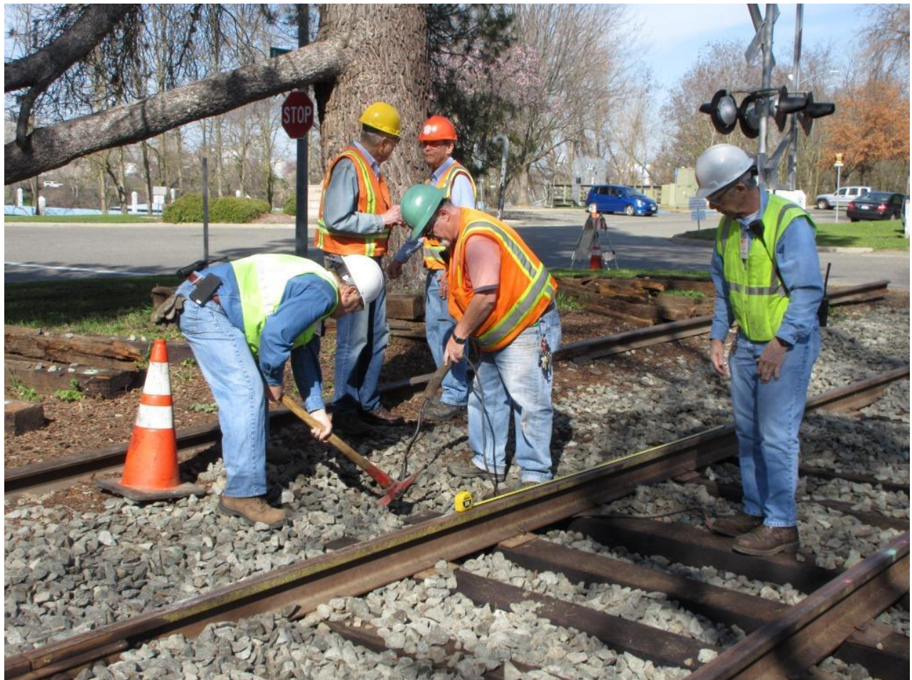
Mike G. digs through the rock to expose the signal wire as Al takes it in hand
