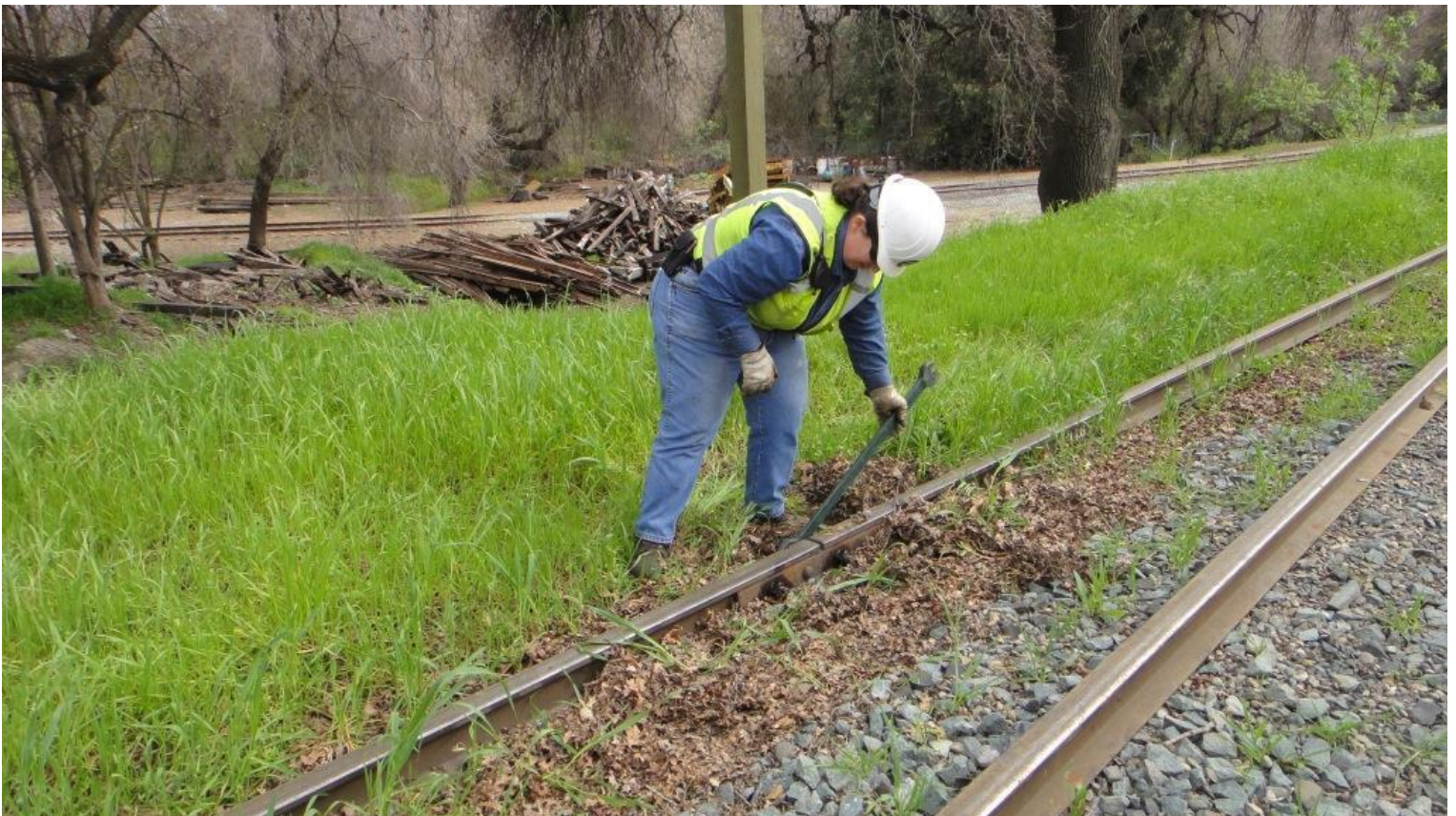
Meanwhile, Heather, working in her natural habitat amongst the weeds, takes apart a rather stubborn joint on the old 75-pound rail
