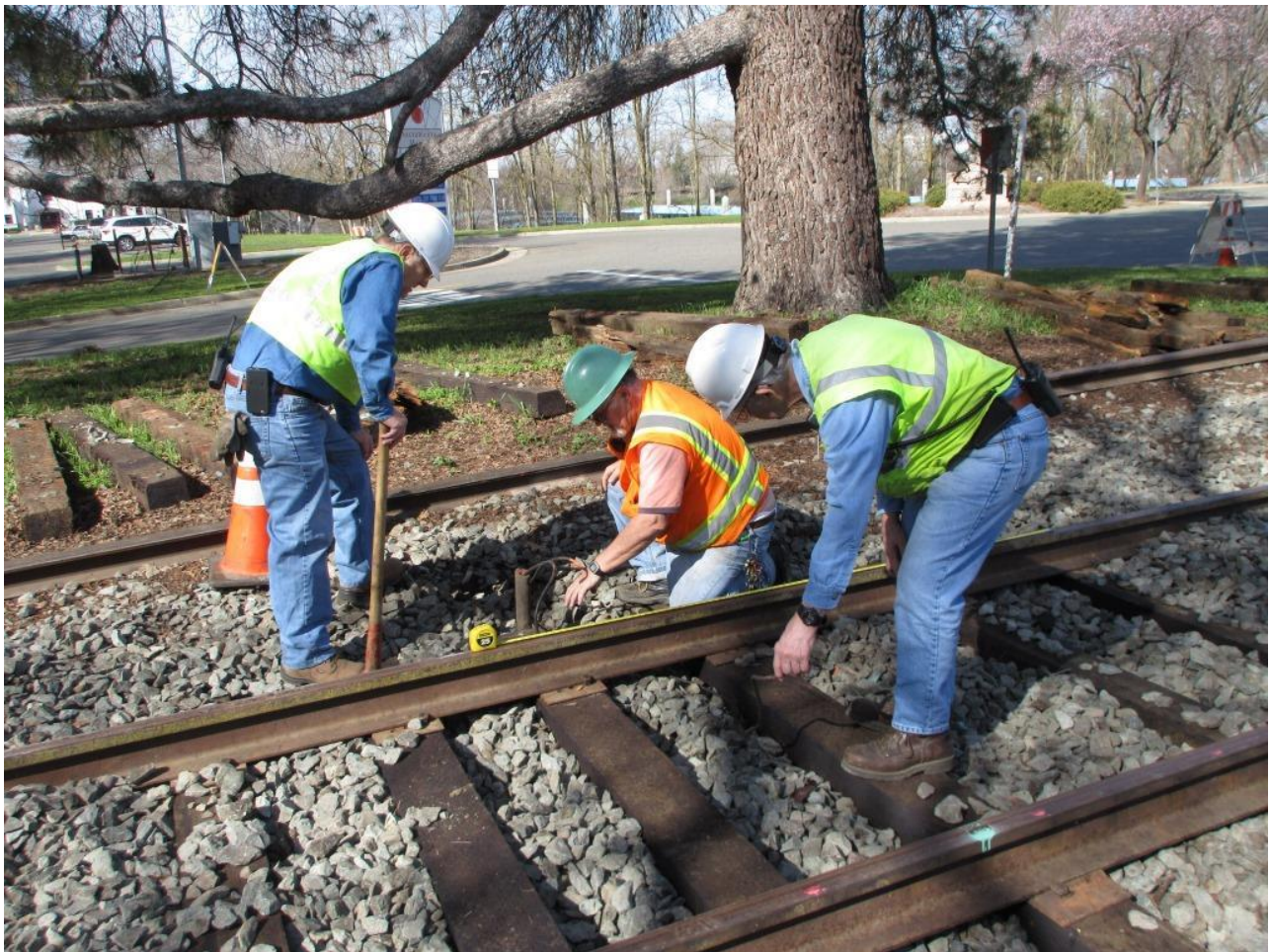
Mike G., Al, and Jim stretch the signal wire to connect to both rails
