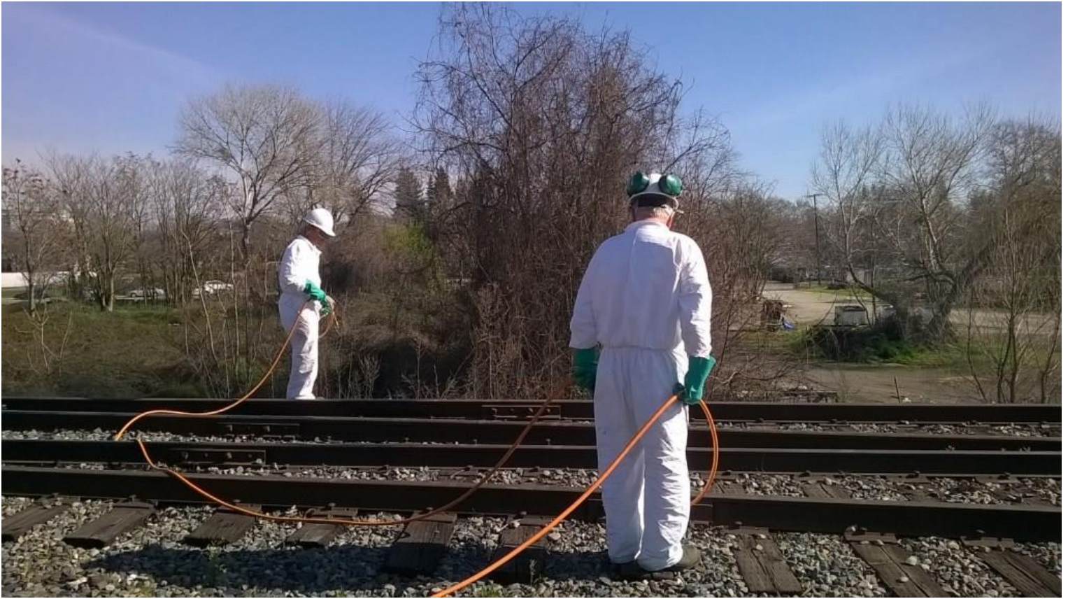
Hermetically sealed, Mike T. and Joe launch counter-measures against the weedy foe at Clunie
