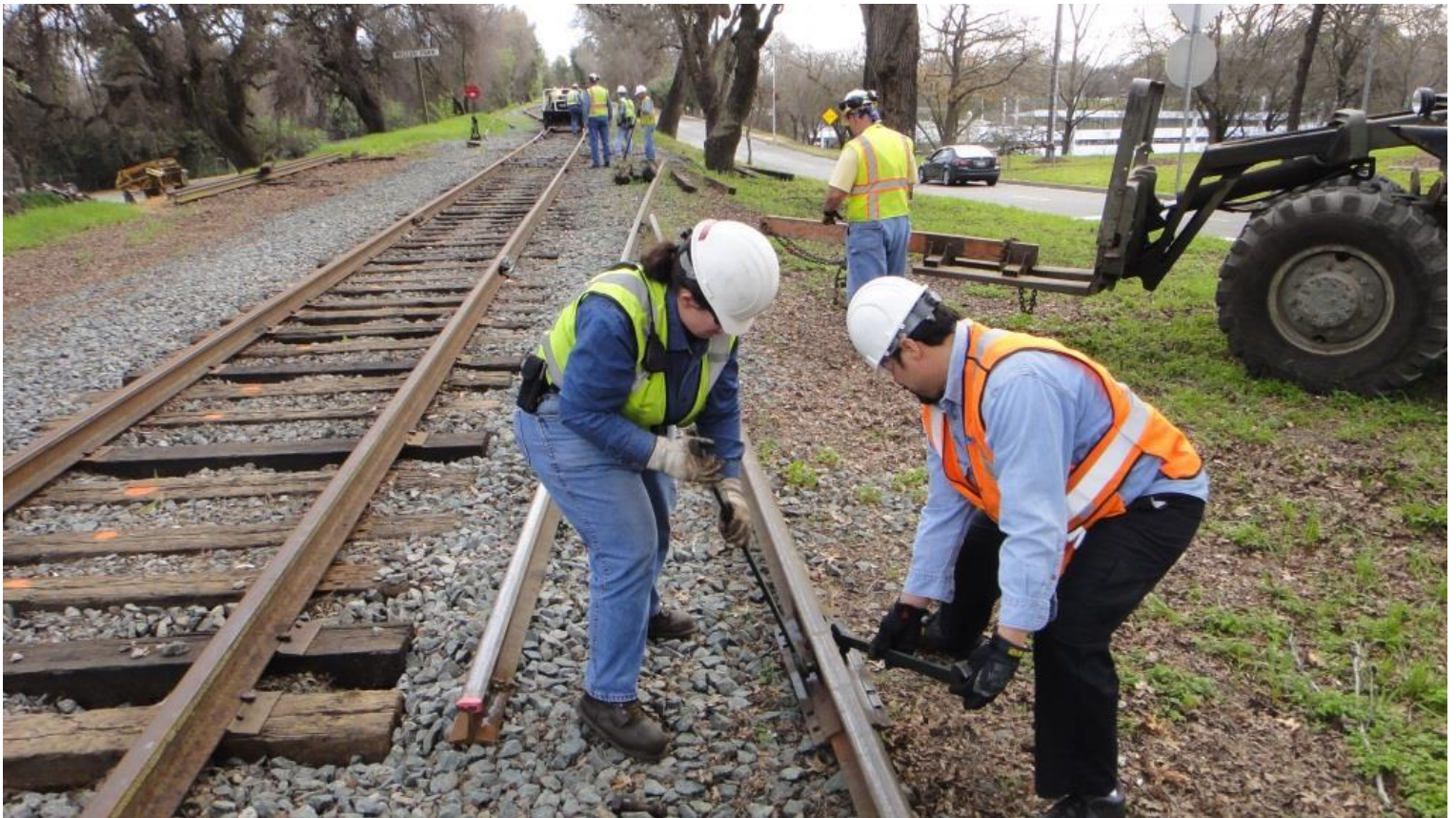
Heather and Jose team-up to take apart a joint on the old 75-pound rail
